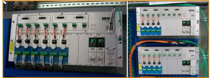
Photos show the RM100 in both rack and surface-mounted installations.
